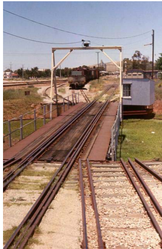
Triple gauge symmetrical (Note the standard gauge thin railhead)
