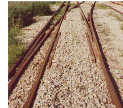
Divergence: (3 gauge) to (b.g+n.g) Main & s.g. Branch. No blades
