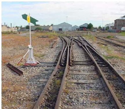
Turnout: (3 gauge) - Main and Branch. 4 moving blades
