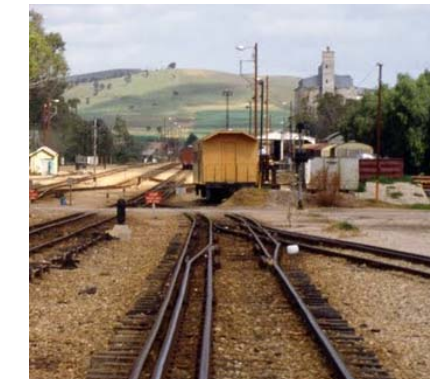
Transition: (3 gauge - common rail) to (3 gauge 'gauntlet')
