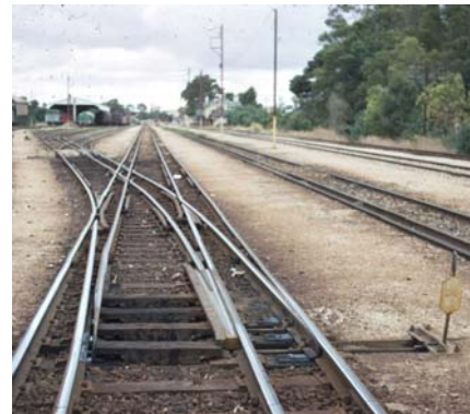
Turnout: (3 gauge) to (b.g+n.g) Branch. 2 moving blades
