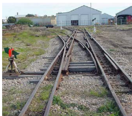
Turnout: (3 gauge) Main to n.g Branch. 1 moving blade
