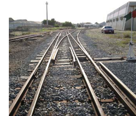
Turnout: (3 gauge) to b.g Branch. 1 moving blade
