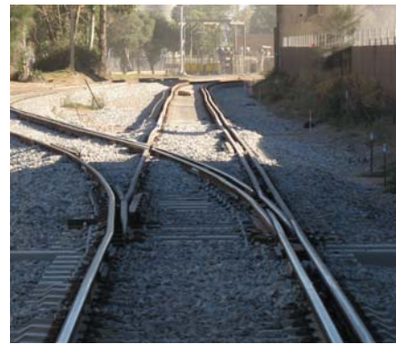
Turnout: (b.g+s.g) - Main and Branch. 3 moving blades
