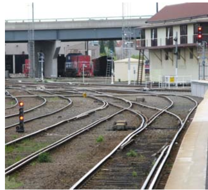
Transition: (b.g+s.g) Conventional transitions (both tracks)
