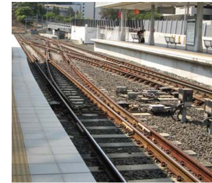
Divergence: (s.g+n.g) to n.g.Main & s.g. Branch. 1 moving blade
