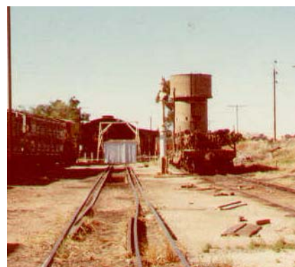
Transition: (b.g+n.g) "3 rail" >>> "Centre line aligned"
