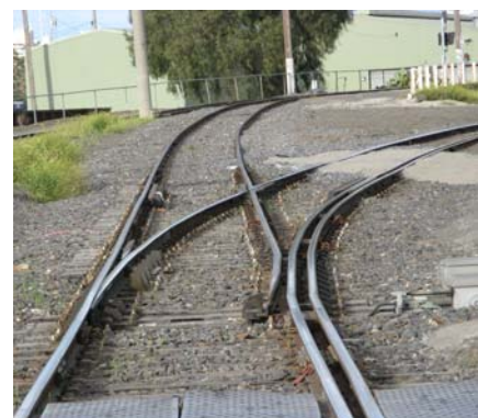
Turnout: (b.g+ s.g) Main to b.g Main. 2 moving blades
