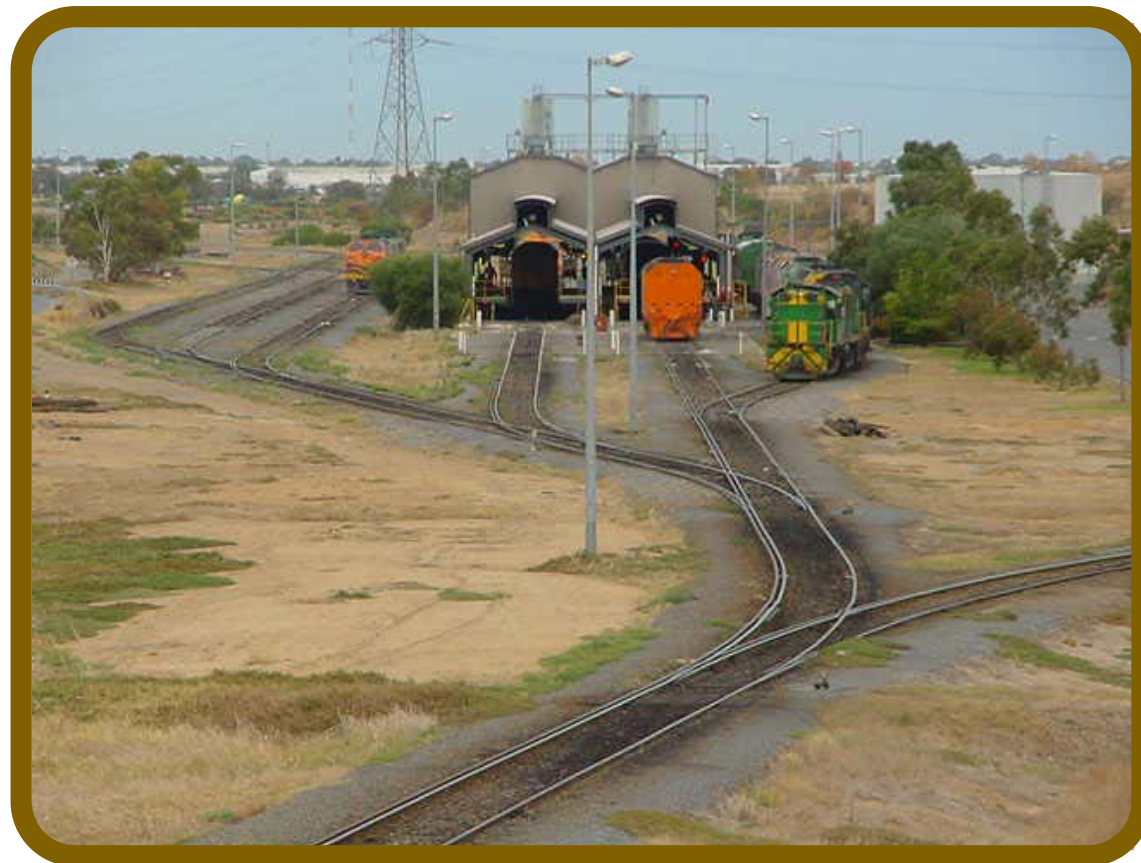
Dual Gauge at Dry Creek MPC
